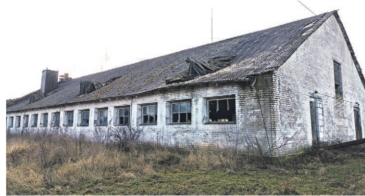
Lammutamisele minev hoone.
